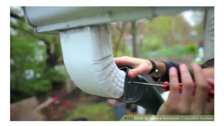
**5.** Place a filter just before the water drains into the tank to prevent debris and leaves from entering
