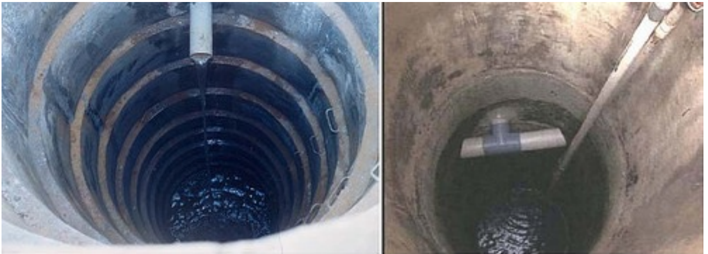
Abandoned Dug Well fitted with RWH Mechanism
