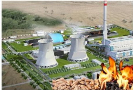
Bagasse Power Plant
