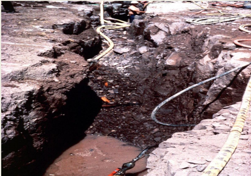
Shear Zone-Backfilled by Concrete
