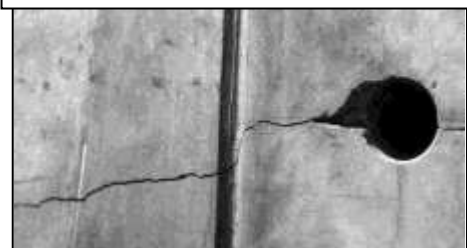
Photo 2 – Cracks in gallery
