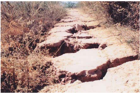
Fig. 18 : Transverse Cracks in Dam
