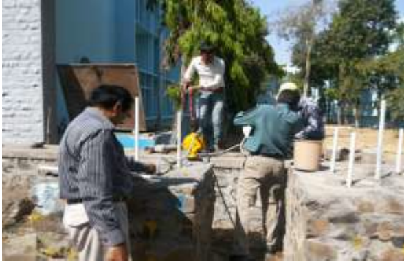
Photos 14 & 15 – Grouting in trial blocks and extracted core after grouting
