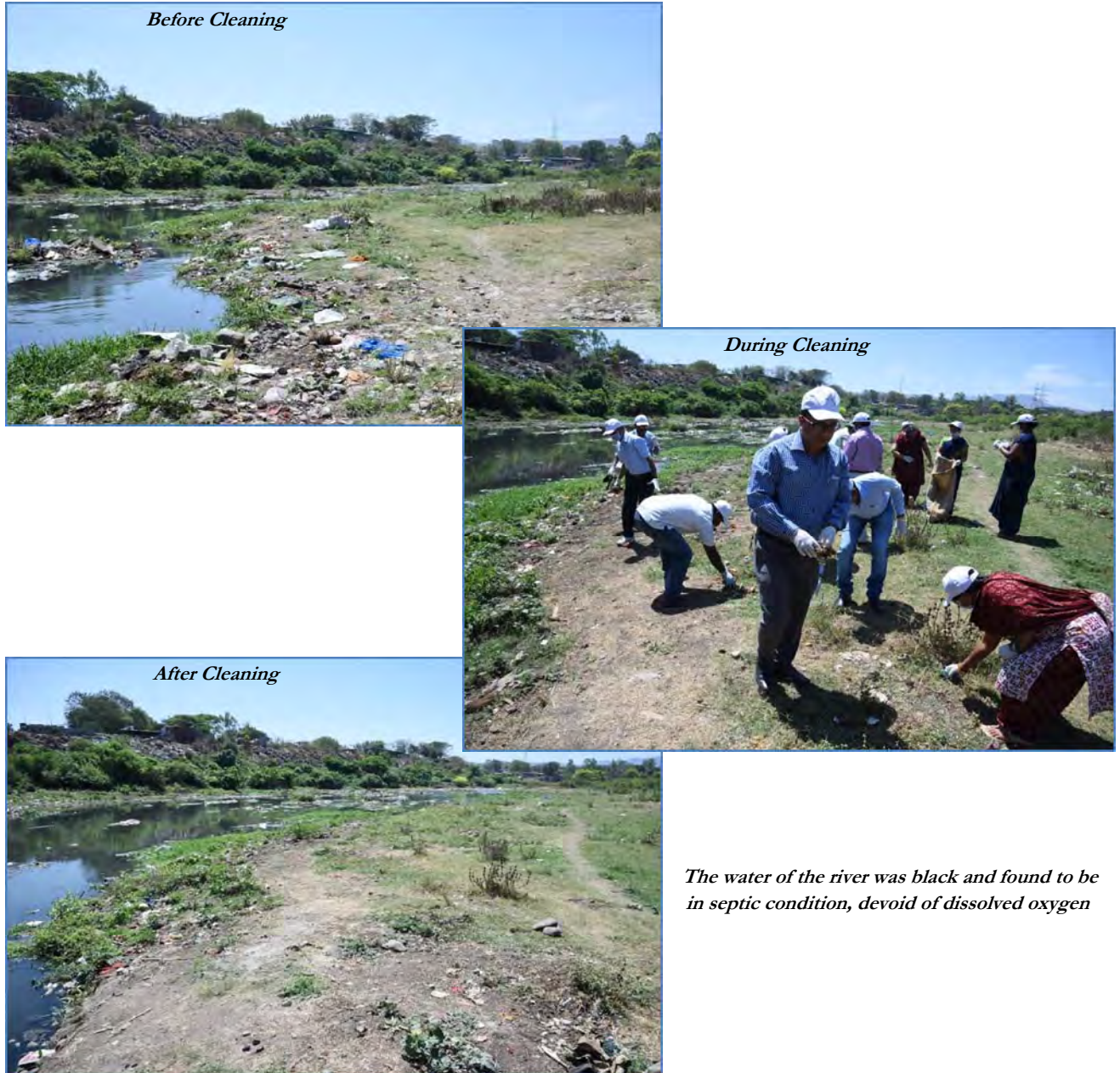
Figure 3. De-cluttering of Left Bank of Mutha River (21.03.2018)
