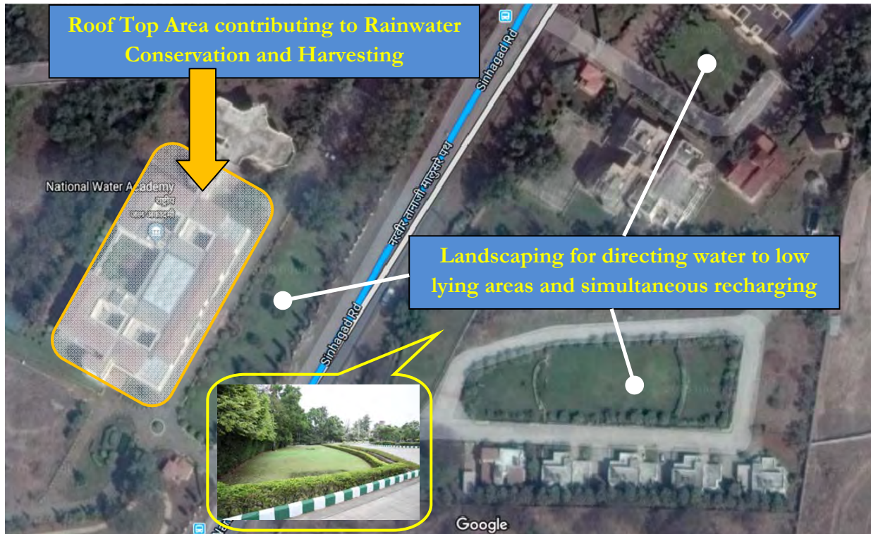
Figure 7. Rainwater Harvesting System
