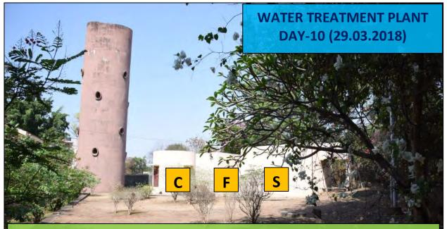
Figure 15A. In NWA, the regular Water Supply (from CANAL) is treated in the Sedimentation chamber (S), Sand Filter Bed (F) and Chlorination unit (C) before being pumped in the Overhead Tank. Treated water is checked for Water Quality and used for all day to day uses. Reverse Osmosis Units treats this water further for drinking purpose.
