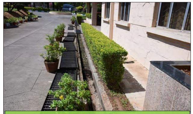
Figure 8A: Silt, dirt and dried leaves had clogged the NWA Campus Storm Water Drains thereby reducing their capacity resulting in water logging during torrential rain.
