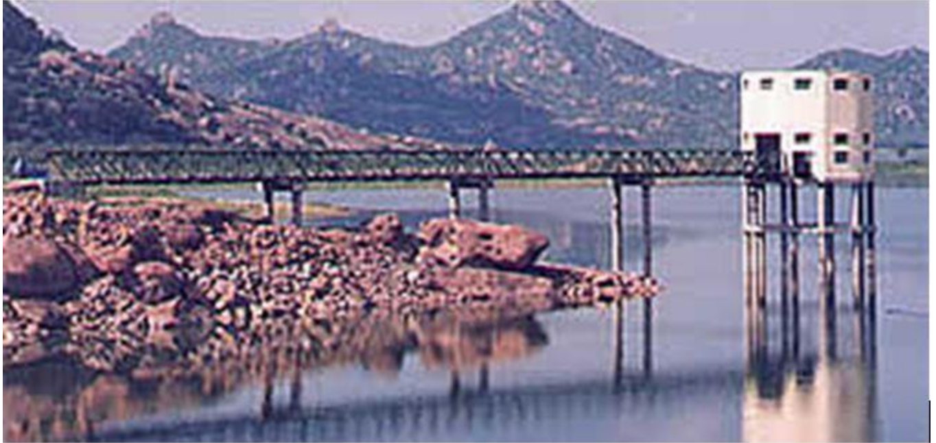
Dharoi (Gujarat) Intake Structure.
