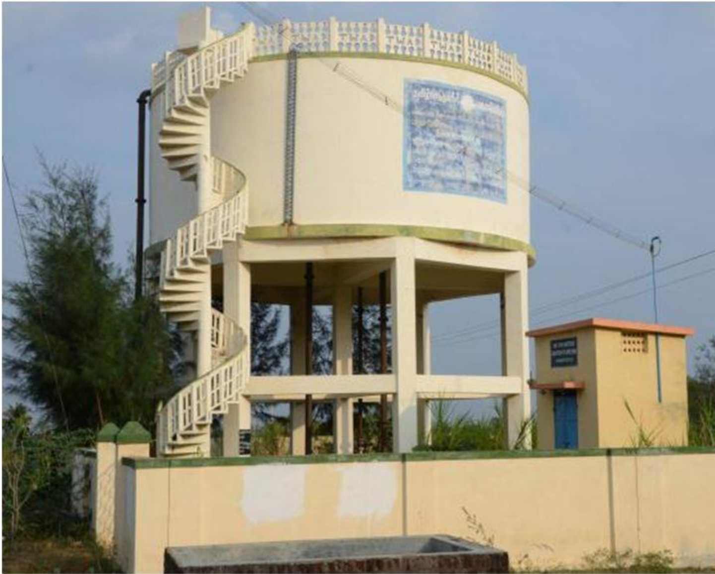
An Overhead Water Tank
